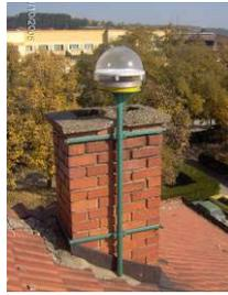
Fig. 8: Type 2 – Pedestal on the metal console
