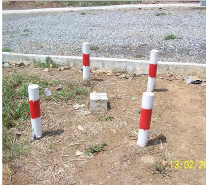
Figure 2 - Reference Marker protected with stakes
