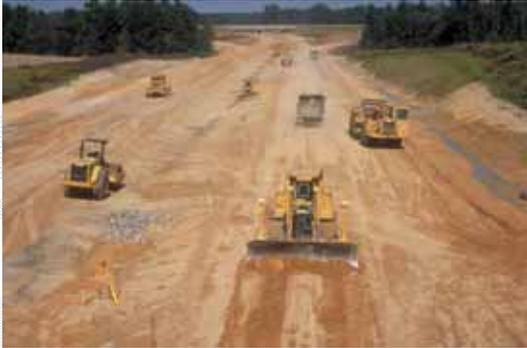
Enables adoption of stakeless construction with machine control systems
