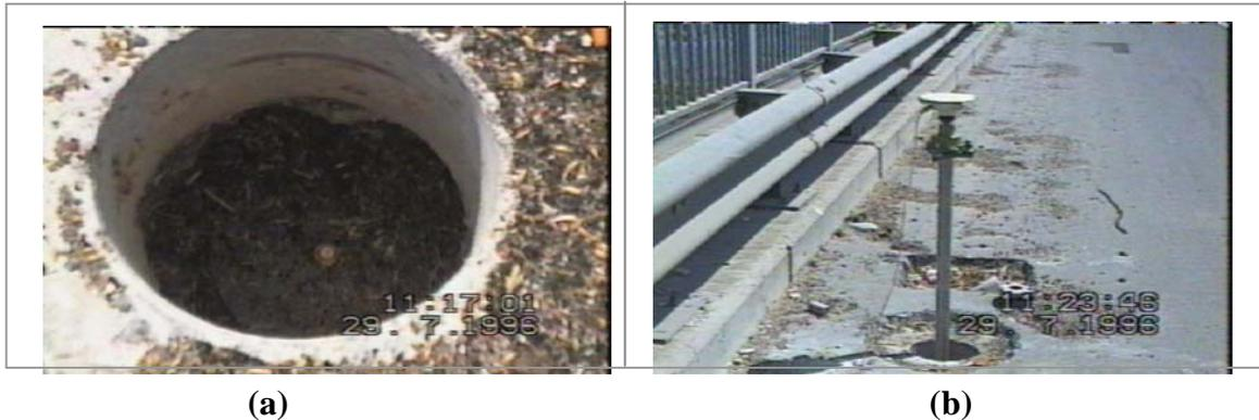
**Figure 1 :** In (a) one of the 24 deformation points established on a pier of the viaduct is shown, in (b) also one of these points is seen during the GPS session.
