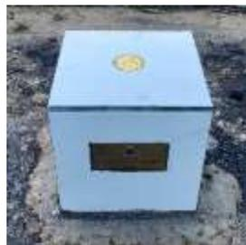
Figure 6. Benchmark Pillar HP.64.09.046 in PT SGP
