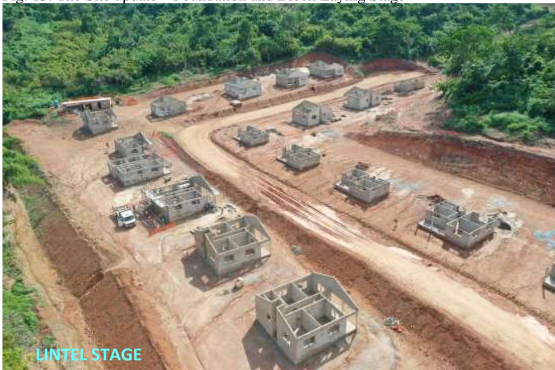
Fig. 14: The site update – Building Lintel Stage from Drone image
