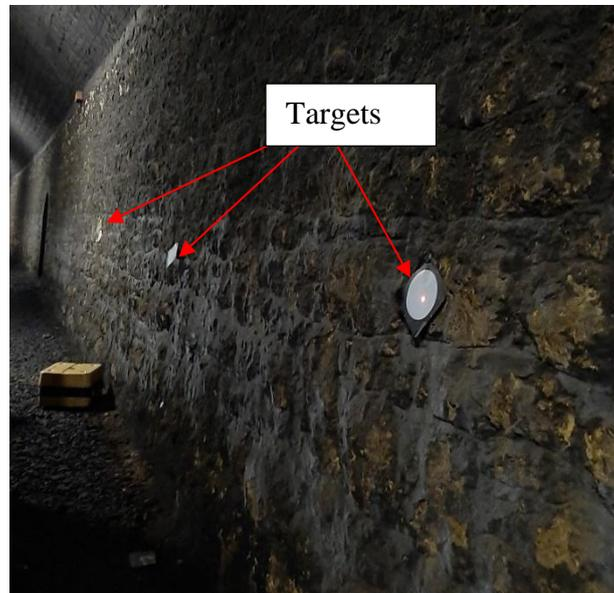
*Figure 5 Targets fixed to redundant service fixings (Anderson, 2022)*
