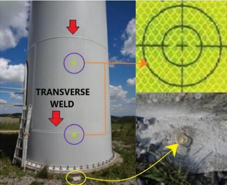
Figure 06 - Object points materialized by reflective targets, pins with semi-spherical head and transverse welds.
