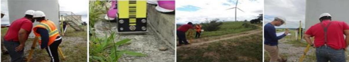
Figure 05 – Geometric leveling performed around the towers and between the two towers.
